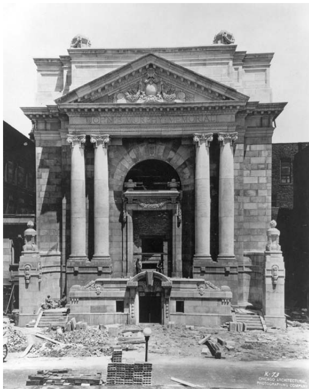
Construction on the Murphy Memorial's elaborate Bedford limestone façade and opulent interior continued for over two years. The photograph at left shows construction progress in July 1924. The photograph at right shows the completed memorial building sometime after 1926. Source: (left) Neenah (Wisconsin) Historical Society, (right) Chicago Architectural Photographing Co. Collection (Erie Street, Folder 221, Sheet 7), University of Illinois.
