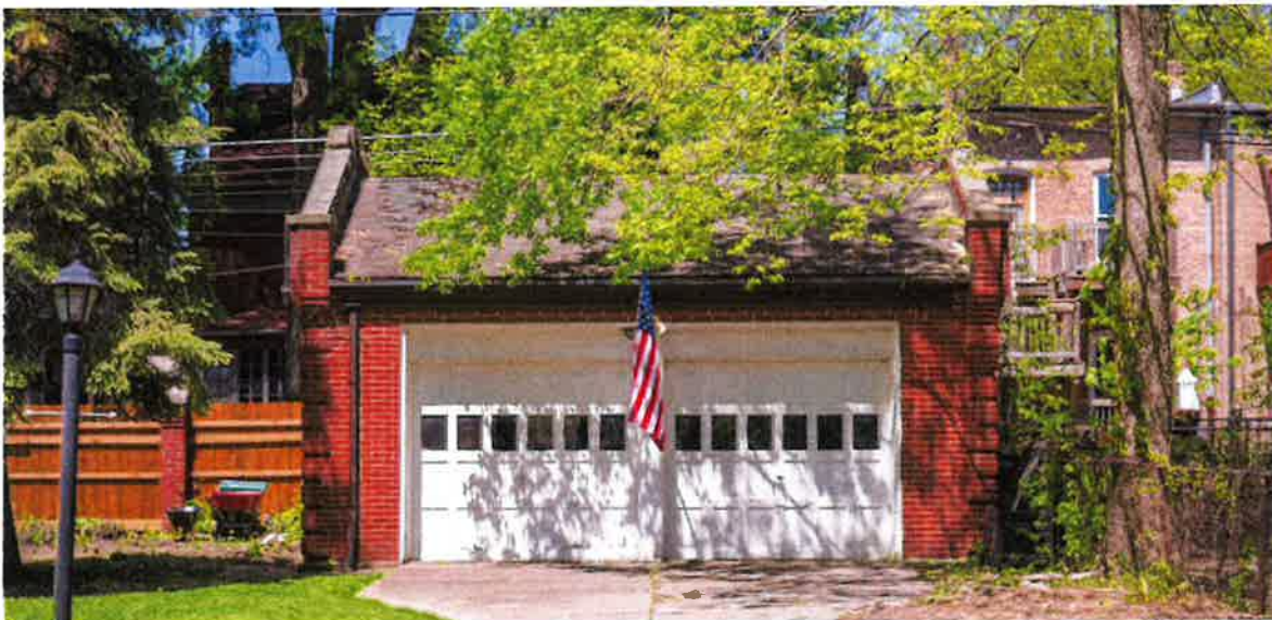
Below: The detached garage at the northeast corner of the lot is closely based on the design of the home. (Photo by Patrick Pyszka)
