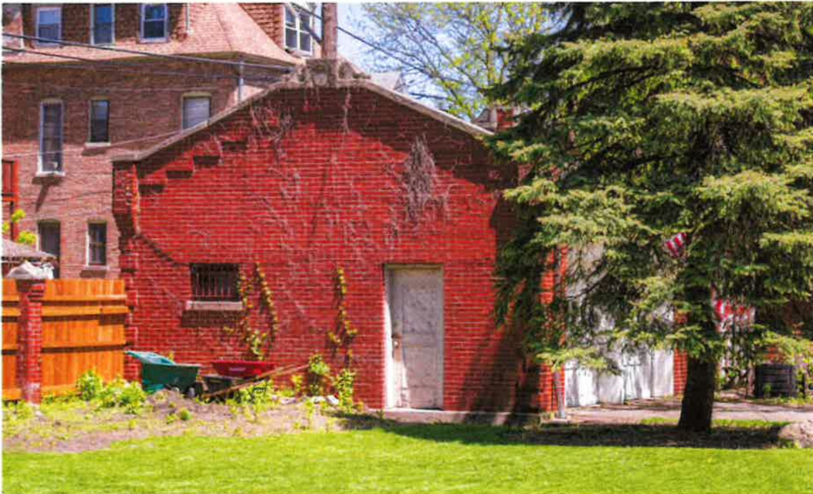
Below: West elevation of the garage. (Photos by Patrick Pyszka)
