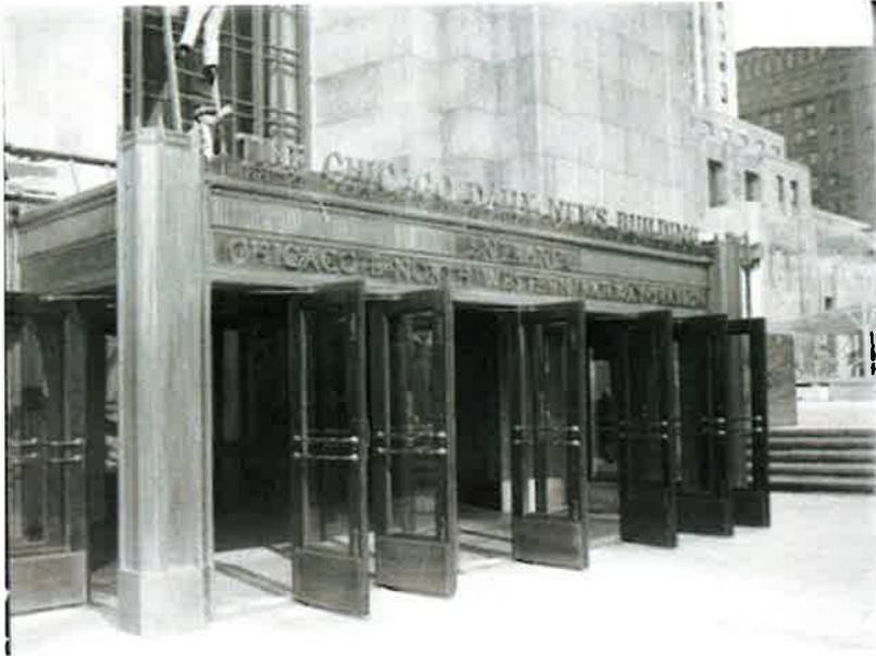
Left: Exterior vestibule at the plaza's south pavilion. The sign extending above the parapet reads "Chicago Daily News Building" and below that "Entrance" and "Chicago & North Western Railway Station." This photo was taken c. 1929 shortly before the dedication ceremony and there are two workmen atop the vestibule still readying the building, one on a ladder leaning against the cast iron window frame. (Source: DN-0089219, Chicago Sun-Times/Chicago Daily News collection, Chicago History Museum)
