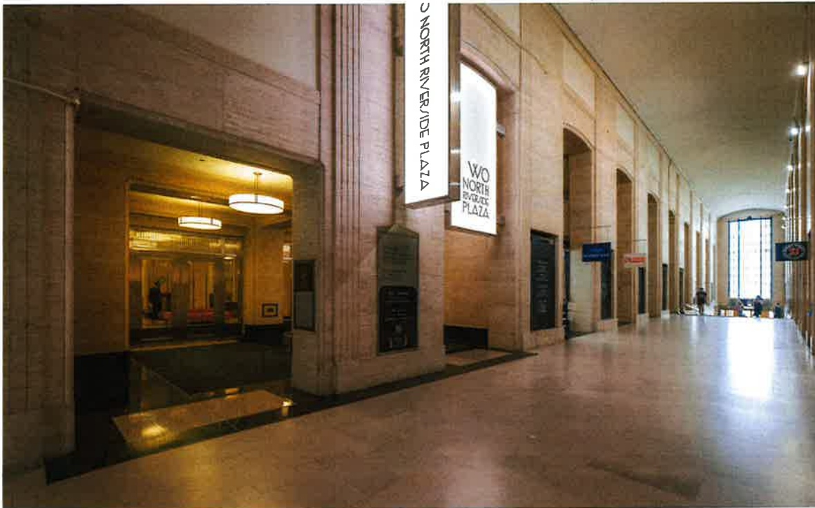
Looking east along the double-height concourse clad with travertine marble. Floor-to-ceiling wall sections edged with stepped profiles emphasize the height of the space between the arched openings. Opening returns have “capitals” with geometric designs. (Photo by Patrick Pyszka)
