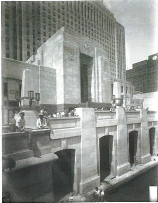
Looking northwest at the south pavilion of the Chicago Daily News Building plaza with the riverfront arcade below, c. 1929. (Source: DN-0020222A-LG, Chicago Sun-Times/Chicago Daily News collection, Chicago History Museum)
