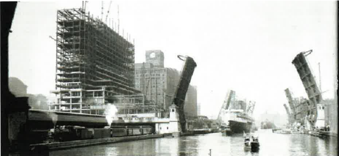
Above: The Chicago Daily News Building under construction, c. 1928. The building was notable not only for its Art Deco design, but as the first major office building in Chicago constructed using air rights over railroad tracks. At left, a train at exits from under the building and plaza, the city's first privately built public plaza for an office building and one facing the river, a rarity. (Source: DN-0086512, Chicago Sun-Times/Chicago Daily News Collection, Chicago History Museum)
