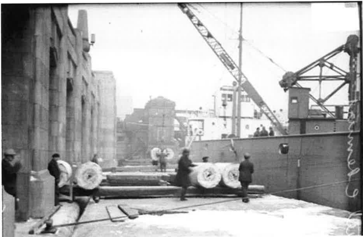
Massive rolls of paper are unloaded off a cargo ship via crane at the riverfront arcade. An elevator was to bring the rolls down below the railroad tracks underneath. According to an Architectural Design article at the time, there was a "conveyor operated through the tunnel under the rows of tracks" which would have been used to get these rolls to storage. Paper and other materials could also be received by truck via a private driveway which ran from Washington to Madison or by train via a private rail spur. (Source: FN-0090137, Chicago Sun-Times/Chicago Daily News collection, Chicago History Museum)
