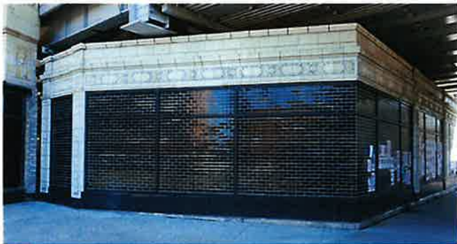
✗ Figure 41. Unacceptable example of a facadectomy as the facade has not been integrated into a new development, but left as an unoccupiable portion of a building and the storefront infilled with brick and a fake storefront frame
