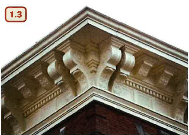
✓ Figure 32. Acceptable substitute material: glass fiber reinforced concrete (GFRC) for terra cotta
