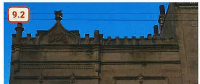
Figure 53. Examples of existing cornices in the district
