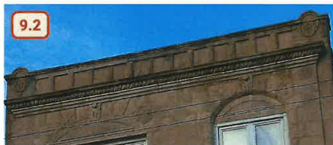
Figure 52. Examples of existing cornices in the district
