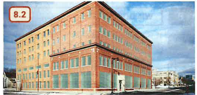
✓ Figure 51. Acceptable example of how window openings were sensitively added to the primary facade as part of the building's reuse
