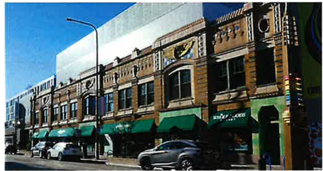
✓ Figure 42. Acceptable example of a facadectomy
