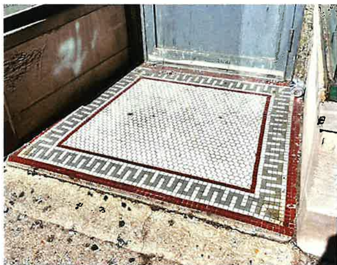
Figure 183. Acceptable example of historic storefront flooring
