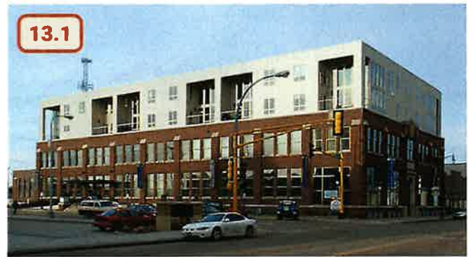
✗ Figure 60. Unacceptable example of a design for an addition to an existing building due to incompatible materials and design of fenestration/recesses (Loopnet)
