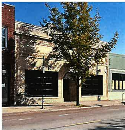
Figure 163. Enframed window wall
