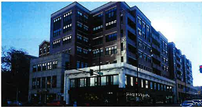
✓ Figure 40. Acceptable example of a facadectomy
