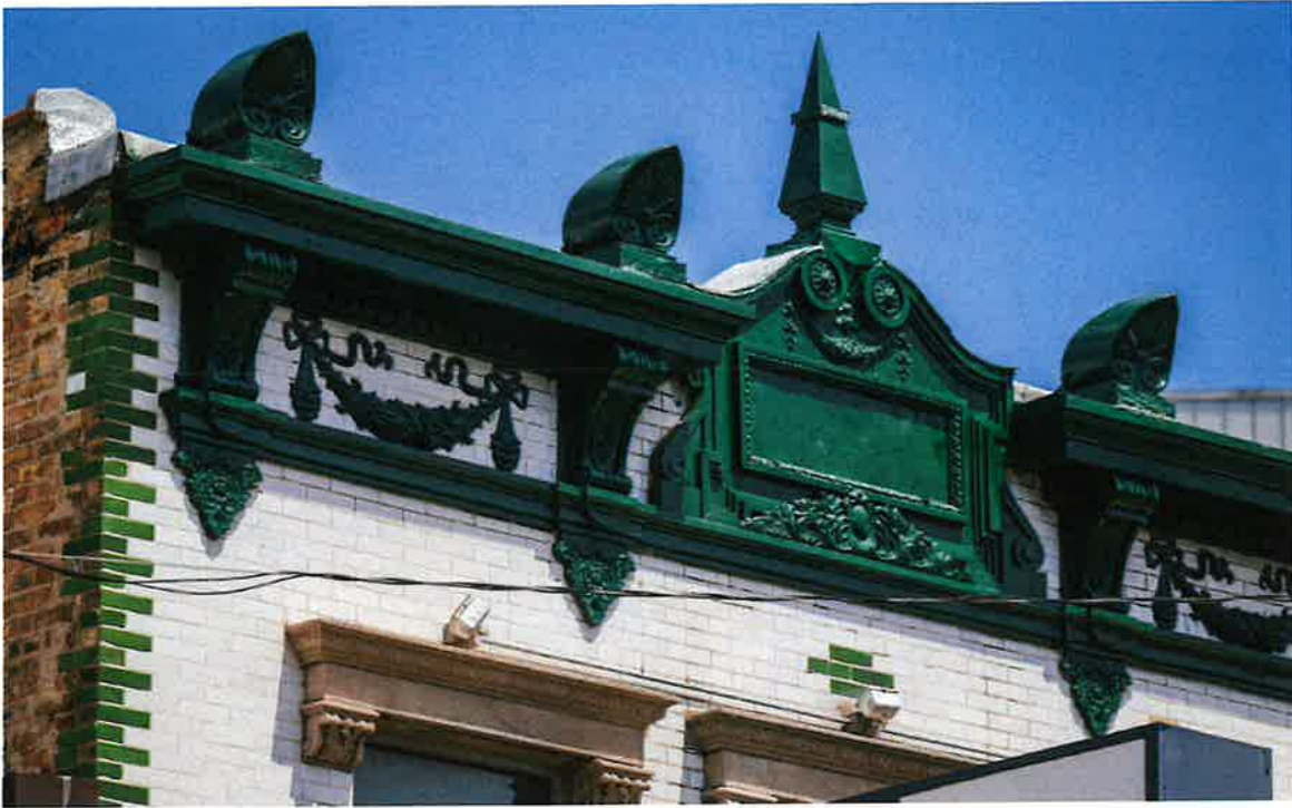
Above: The front façade is topped with a pressed metal cornice of unusual size and ornamentation for this building type. (Photo by Patrick Pyszka)
