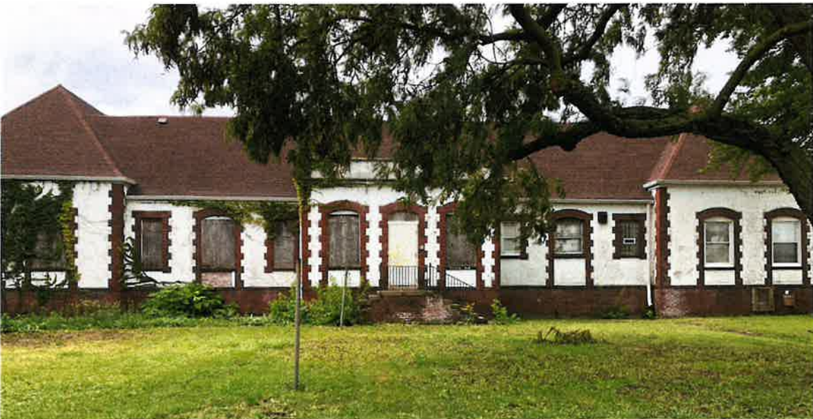
The east elevation of the dormitory.
