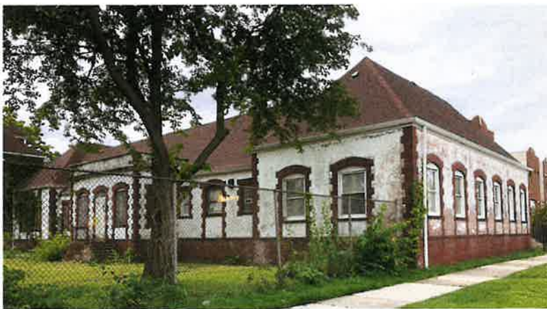
The dormitory at 2678 West Washington Boulevard.
